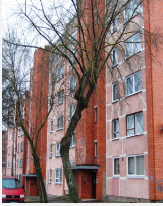
Tautas Street 30, Daugavpils, was one of the buildings audited
